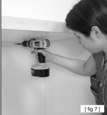
After glue is dry locate studs in wall (fig. 7A). Attach cabinet to wall using 2 1/2" screws (fig. 7). **STACKING CABINETS:** If you are stacking the cabinet place cabinet on top of already installed cabinet, carefully overhang cabinet to revealing dowel holes. Push dowels into all of the pre-drilled holes (fig. 7B and 7C). Next align dowels with cabinets below (fig 7D). Set cabinet down in place and attach to wall (fig, 7).
