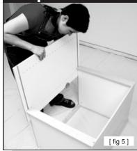
attach to face frame and side panels (see fig. 5B and 5C) in the middle of the cabinet. (see fig. 5D)
