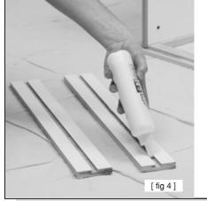
Glue the female dovetail On the nailer see fig. 4. Slide one nailer onto the top shelf (fig. 4A) and one nailer onto the bottom shelf (fig. 4B). Make sure they touch the side panel.
