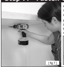
After glue is dry locate studs in wall (fig. 7A). Attach cabinet to wall using 2 1/2" screws. (See fig. 7) NOTE:
